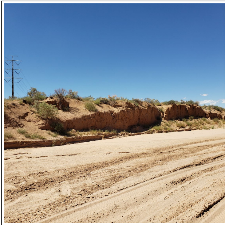
14. Typical Arroyo walls, center portion of Project Area
