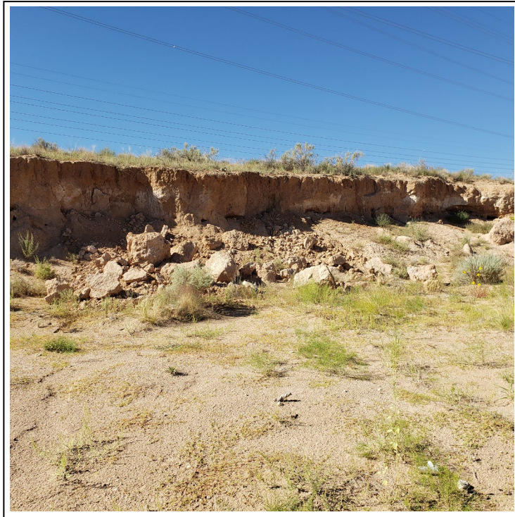
5. Arroyo wall sloughing off
